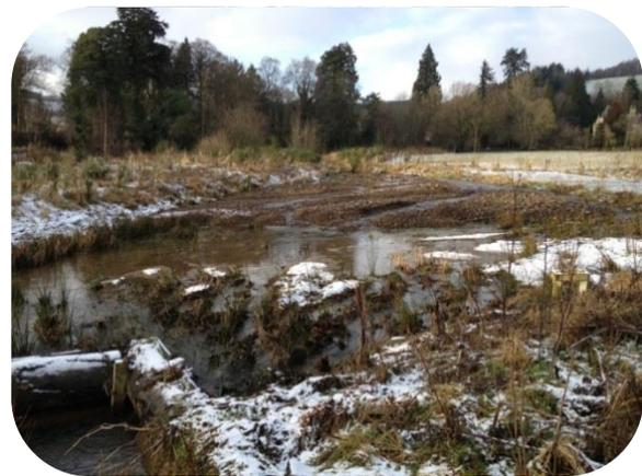
**The designed sediment basin empty in summer 2013 (left); and with gravel/sediment after a high flow event in winter 2013 (right). Photo credits: Selkirk Flood Protection Scheme.**
